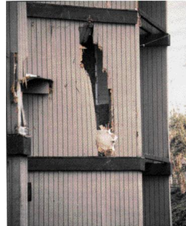
Breach of the building envelope by wind-borne debris.
