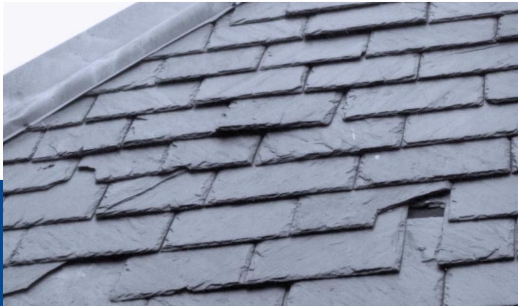
Slate roof damaged by hail.
