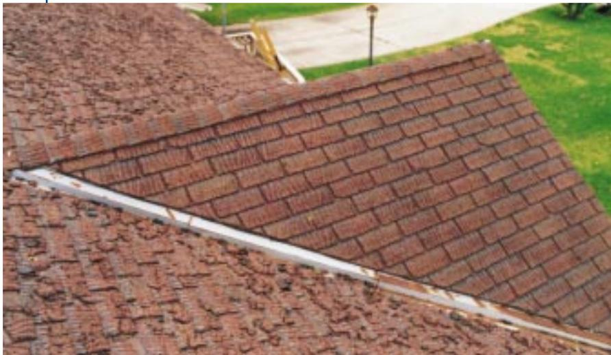
Asphalt roof shingles damaged by hail.
