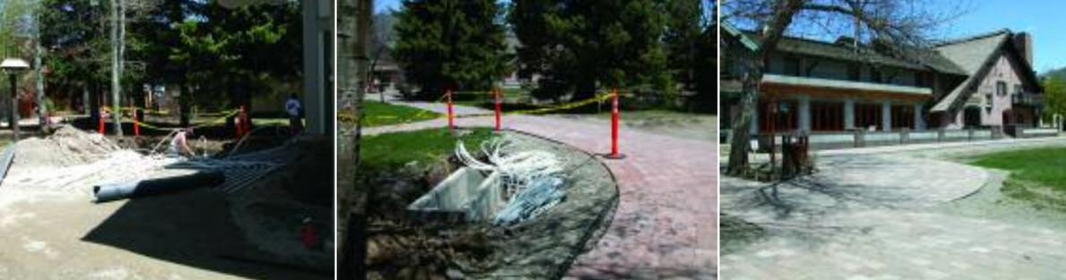
RadiantPex installs in sand below concrete pavers and will join with a manifold. Imagine warm pavers instead of shovels, blades or salt.
