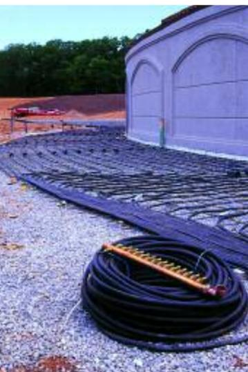
Onix shown in infrared light connected to a manifold.
