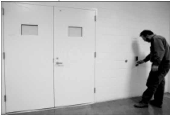
An example of a key-card security system that limits staff access to storage areas. Here, Robert Herskovitz, MHS Outreach Conservation program, demonstrates the key card system in the MHS storage area.
